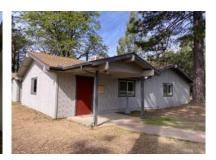
The wood siding and trim located throughout the Clubhouse appeared to be in fair condition without major signs of damage, separation, cracking, or other signs of distress. We have budgeted for 10% to be repaired or replaced every 10 years to coincide with painting.
