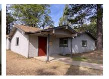
The present condition of the paint on the wood/trim siding was in good condition. There were no areas where the paint was peeling and chipping away. Proper painting intervals will help protect the component underneath from unnecessary damage or from exposure to the elements. Before the buildings are painted, the preparation should include power washing, scraping, sanding and repairs as found necessary.
