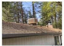
The Composition Shingled roof on the Clubhouse appeared to be in fair condition. There were minimal signs of warping and curling. It's recommended that all roofs over 10 years old be inspected by a reputable roofing inspector and be repaired as indicated.
