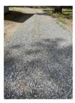
The gravel bladed road located at the Clubhouse is approximatelly 916 feet long and 10 feet wide. The road appeared to be in fair condition; no noticeable or troublesome erosion was apparent on or through the gravel roadway. Annual inspections and weed control is recommended. It is best to correct any damage or abnormalities as quickly as possible to prevent any permanent or large scale repairs.
