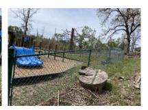
This component covers the replacement of the 4ft thermoplastic covered chain link fencing surrounding the kids area. The fence appeared to be in good condition without major signs of defect.
